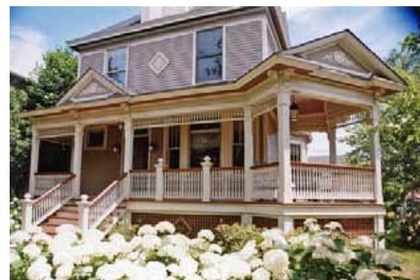
LEFT: On this transitional 1903 house, the diamond ornament is made of pressed metal; note the ornaments, too, in the gables. TOP LEFT: On a Chicago Foursquare, posts on the newly reopened porch are inlaid with mosaic glass, giving the impression of double columns.
