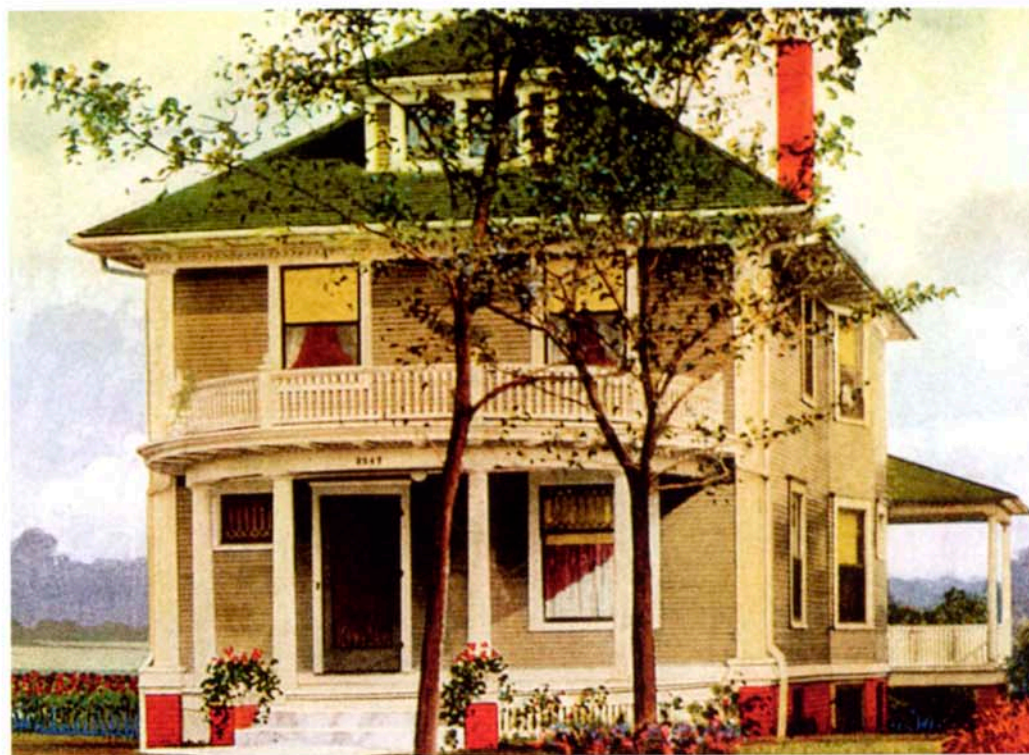
The Colonial Revival-style elements of this American Foursquare are enhanced by the cream-color trim paint on columns, balustrade, and pilasters at the corners. The body color, a soft olive green, lends interest without high contrast.
